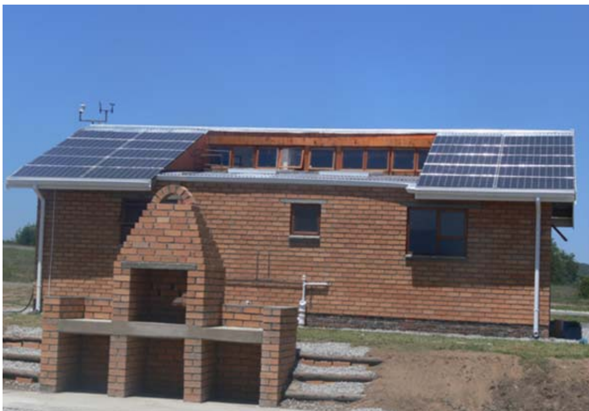
Figure 1. BIPV panels on north facing roof
