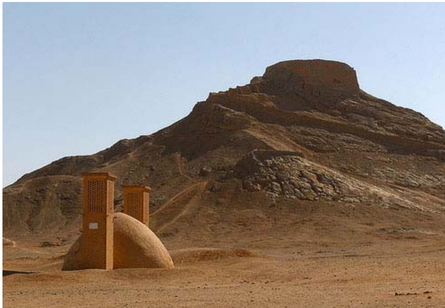
Figure 1. Two-wind catcher cistern (Abar-Kooh's cistern)
